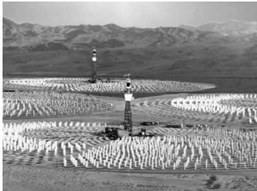
Figure P8-16.1 Solar field design. Five 265-m-tall towers with three heliostat fields/tower, on 275 acres of land in Daggett, CA. Net concentration 3,868 suns and 295 MW delivered to each solar reactor. (Melinda M. Channel, Jonathan Scheffe, Allan Lewandowski, and Alan W. Weimer, November 11, 2009. Also see: Chemical Engineering , 116, p. 18, March 2009).
